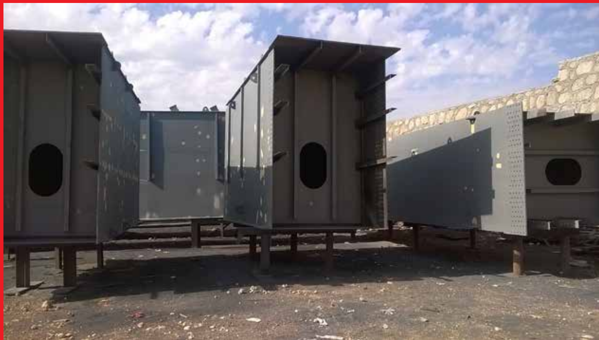
Port Crane Support Columns
