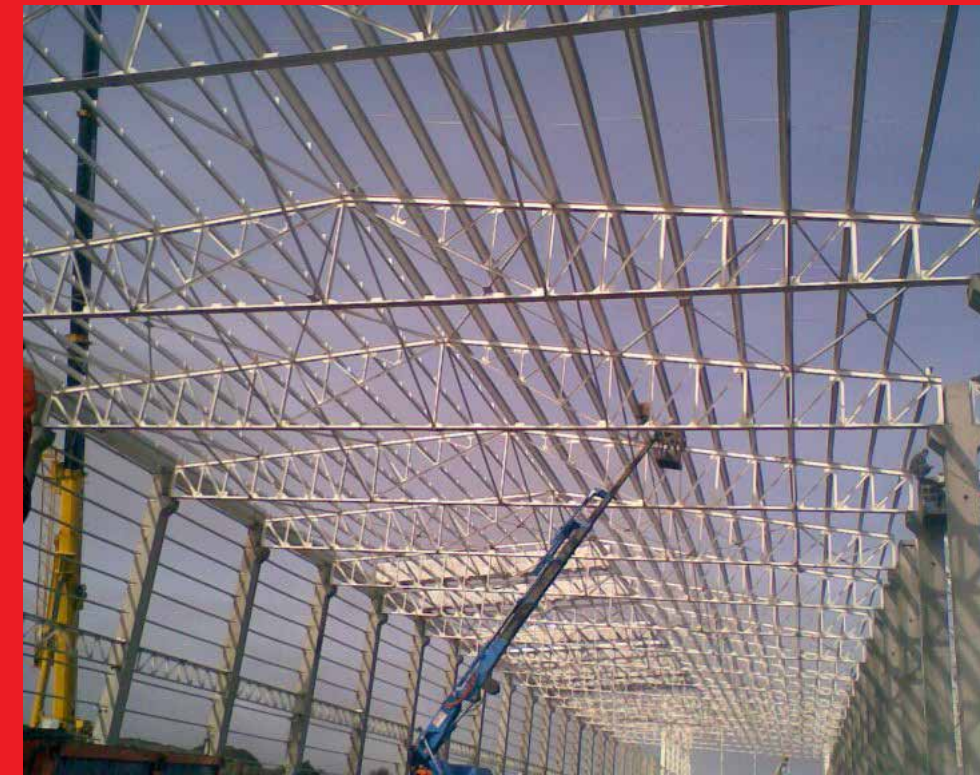
Steel Construction Factory Installation
